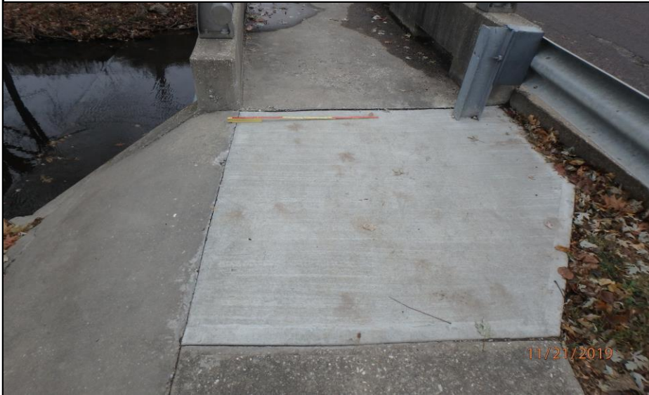
Typical Sidewalk Repair on North Sidewalk - Looking East
