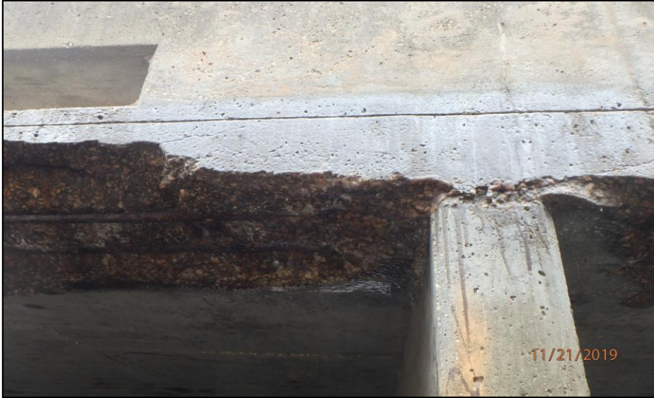
Polyer Overlay at South End of All Cells - Looking North
