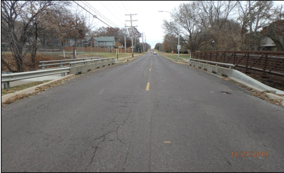
Approach Roadway - Looking East
