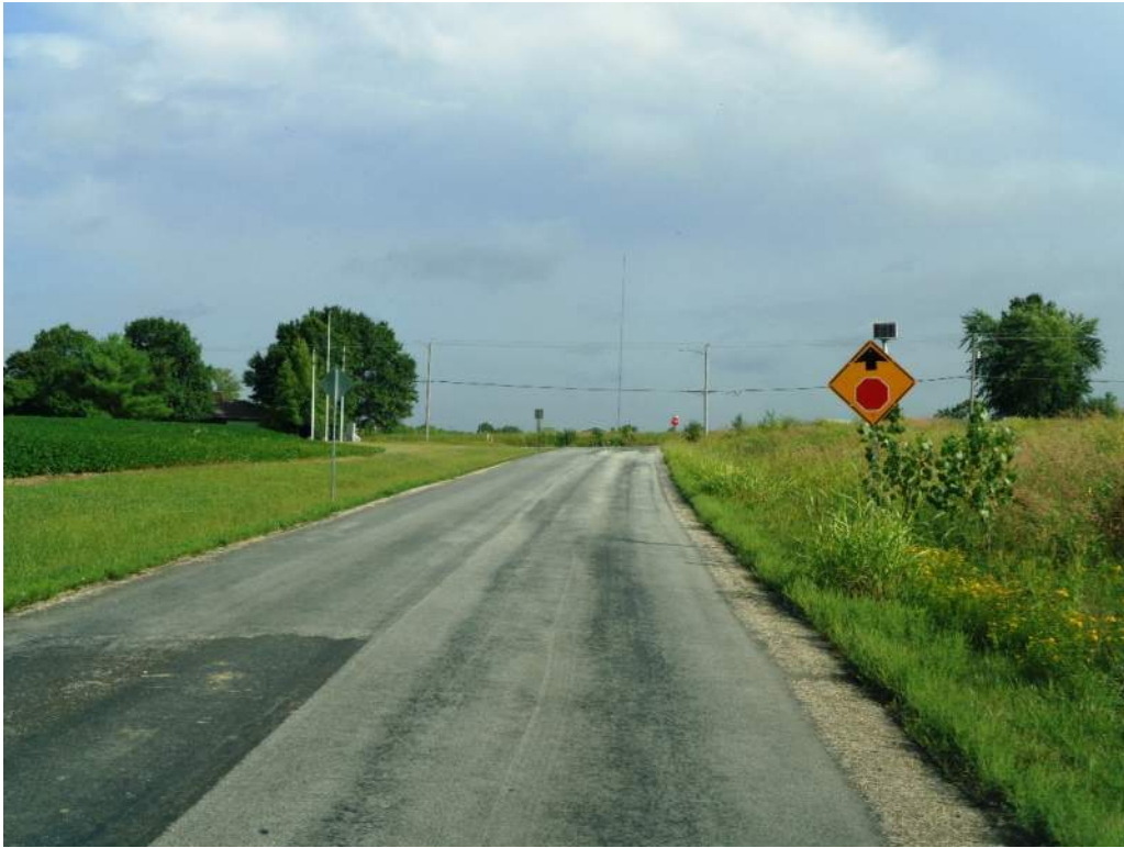
Photo 9: 158 th Street and Parallel intersection, northbound. An advanced warning “Stop Ahead” sign has been installed for vehicular traffic. No pedestrian facilities exist.
