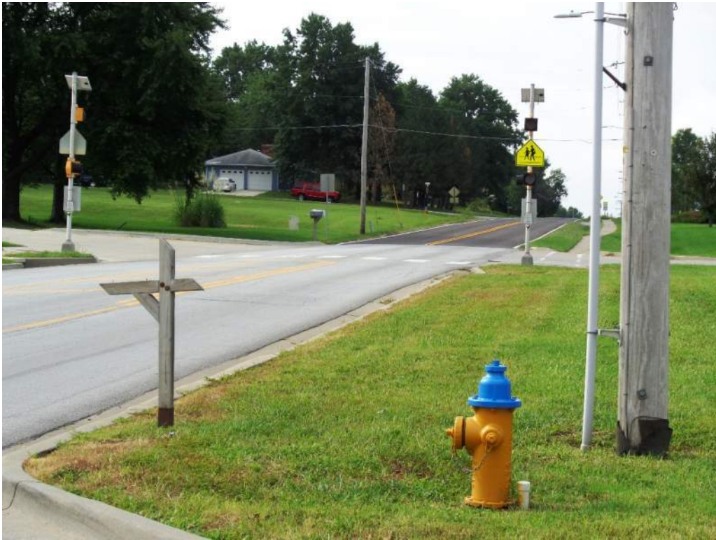
Photo 10: Crosswalk with Pedestrian Warning Signs, Pedestrian Controlled Signal Heads, and Circular Warning Flashing Beacons at 155 th Street, just north of Elm Street.
