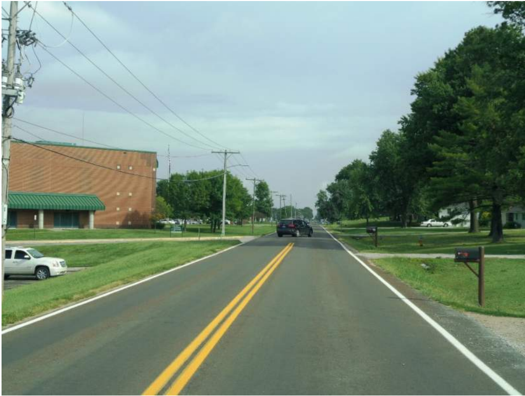
Photo 5: Southern high school entrance, just north of 155 th Street and Parallel Road intersection, looking north. No turn lanes into high school, causing stacking.
