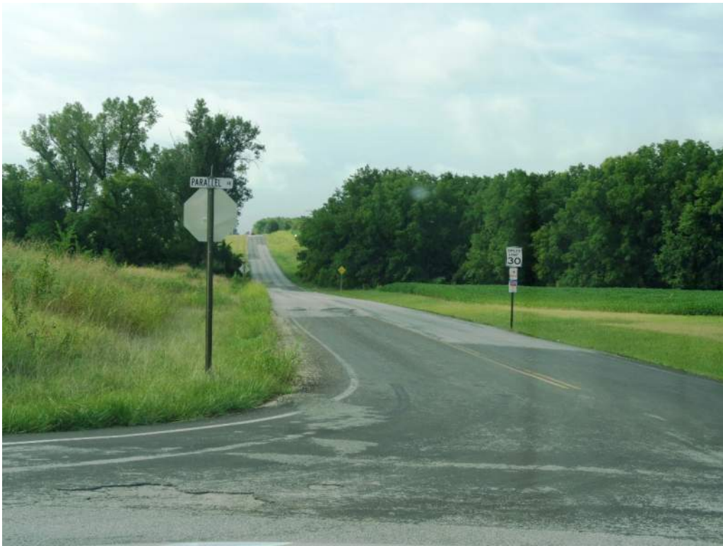
Photo 8: 158 th Street and Parallel intersection, looking south toward library. Northbound traffic is stop controlled. 158 th Street corridor is programmed for substantial development with 350 single-family homes and 64 apartments in process.
