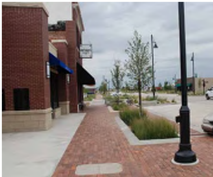
Figure 17 | These photos from Kansas City, MO (top) and Greensburg, KS (bottom) show how green infrastructure solutions can be incorporated into the amenity zone of the street right-of-way.
