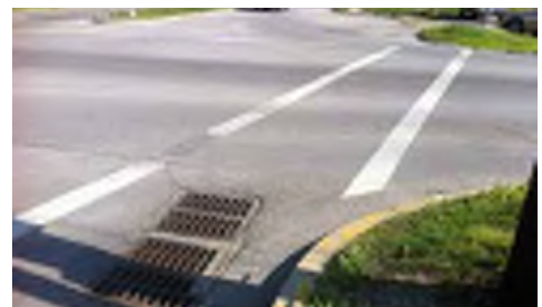
Figure 3 | Top photo: Sidewalk installed in 2012. Second photo: Existing crosswalk. Third photo: Unplanted tree pits. Fourth photo: Only break in sidewalk between Van Horn High School and Independence Square. Fifth photo: Stormwater grate in crosswalk.
