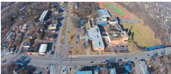
Existing Conditions Images
