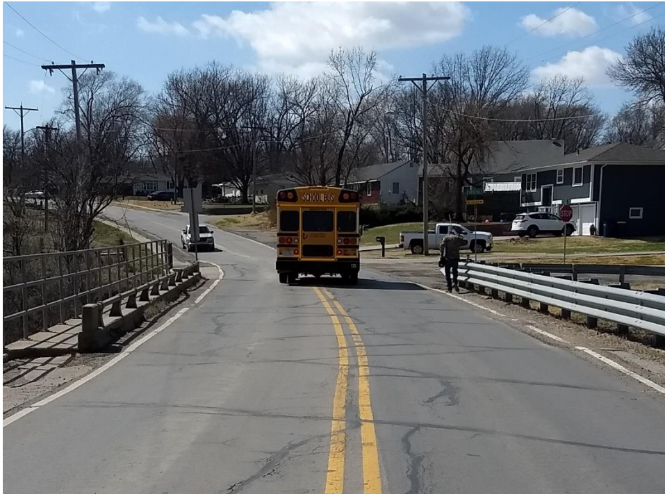
83 rd Street looking west. Pedestrian using the non-sidewalk side of the bridge due to poor sidewalk condition and insufficient lane + shoulder width for the bus to pass safely by him.
