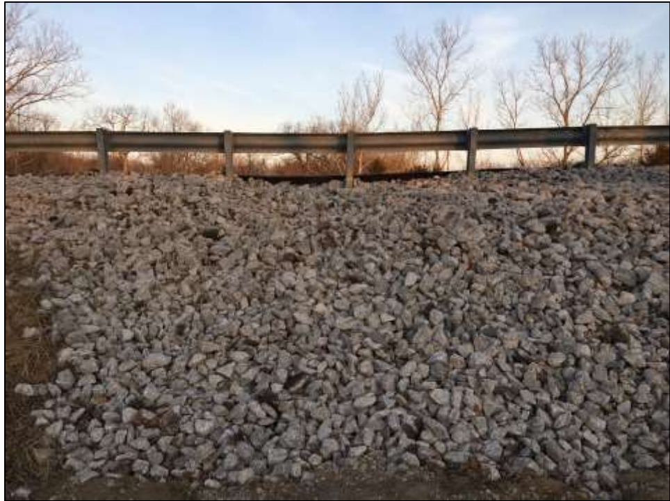
Figure 4 – Photograph of Northbound Raytown Road Fill Slope Protection Source: WSP (March 15, 2018)
