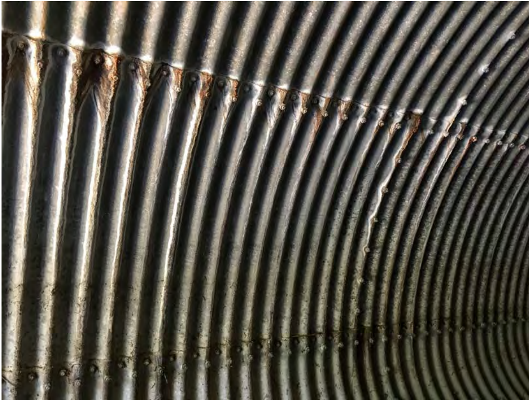
Photo 5 – north face of the north culvert roughly 30' from the upstream end.
