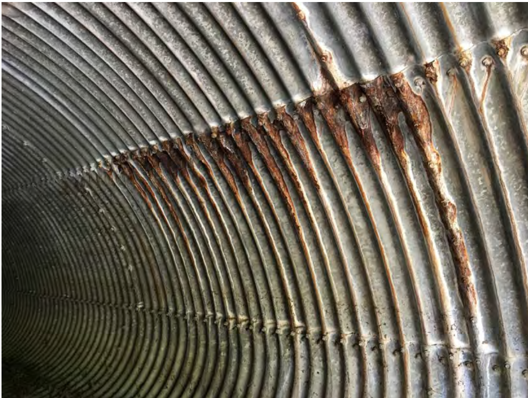
Photo 6 – south face of the south culvert roughly 30' from the upstream end.
